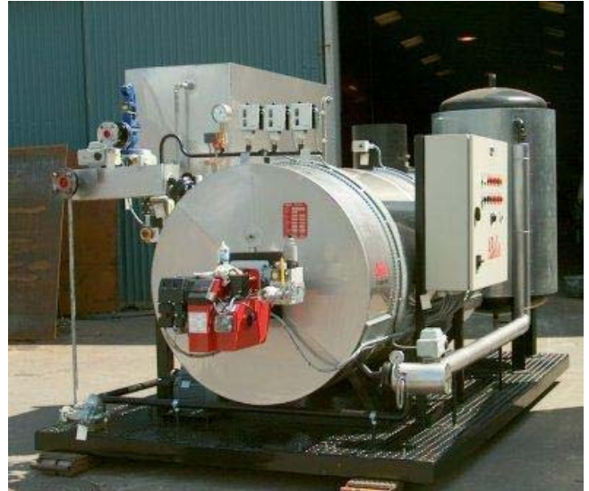
Skid-mounted steam boiler system
